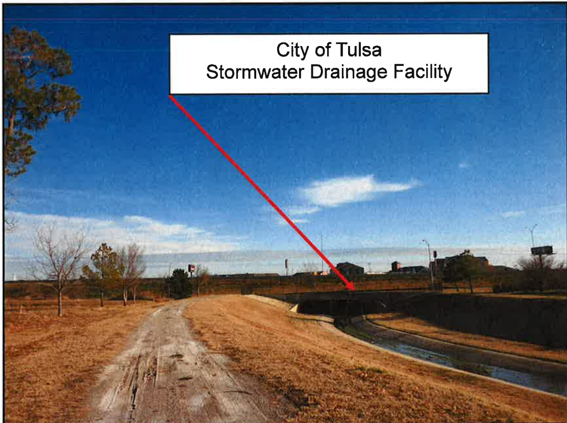
7600 E 31st Street - Looking northeast towards I-44 and Drainage Channel
